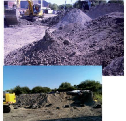
From the heterogeneous to the homogeneous source material (bottom right)
